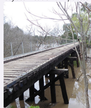
Trestle during floods
